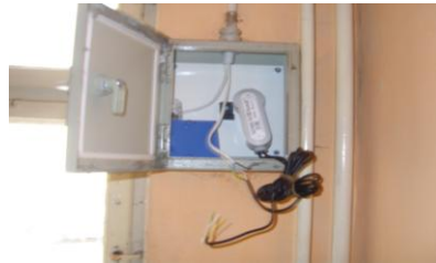
Figure 5. Replacing electronic reader CF M-BUS COMBI network radio module Sensus ((S)) cout-P2 in block staircase [1]
